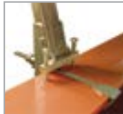
Stanchion installation complete
